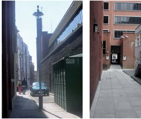
Improve the walkways
